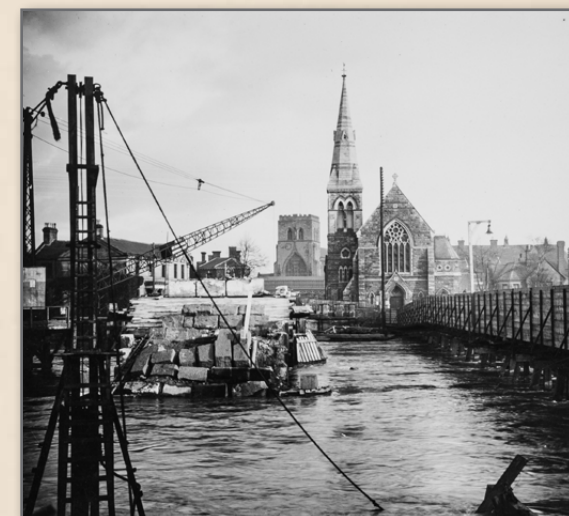
A collapsed arch caused by flood damage during the dismantling of the old bridge on 23 October 1925, with the temporary wooden trestle bridge to the right. Shropshire Archives ref: PH/S/13/E/2/60
