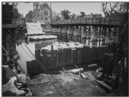
Reconstruction of the bridge in progress, with the temporary trestle bridge to the right. Shropshire Archives ref: PH/S/13/E/2/119
