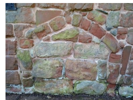
Fig. 4. Blocked squint recess at St John the Baptist, Ruyton, with the open squint placed inside the recess visible internally.
